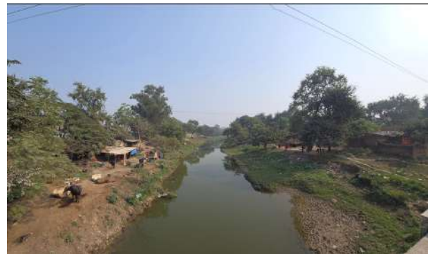
Sone Canal with Encroachments on its channel
